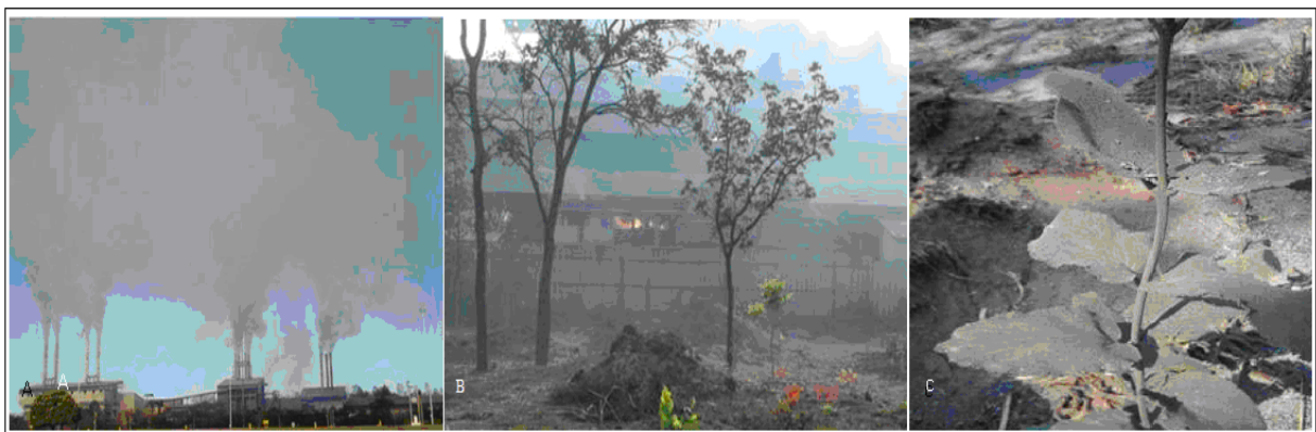
Figure 3. (a) battery of industrial furnaces, homogeneous laminar flow showing the stability of the plume photo made at 9:00 am (height of plume 4 km), (B) diffuse plume, flow, lapse below and inversion – fumigation, (C) examples of plant exposition to the smoke.
